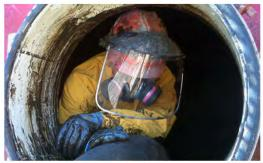
**Confined Space & Vessel Entry** Internal cleaning and coating inspection. Trained and certified personnel to open, purge, and monitor air quality, clean residues, and perform visual inspection. Complete safety supervision and cascade air units with SCBA's available.
