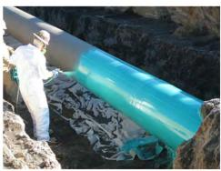
**Pipeline Coating and Reconditioning** Trained and certified personnel to meet all DOT -OPS Operator Qualification requirements to perform sandblasting and coating on pipelines and associated facilities. All work performed in with NACE and SSPC
