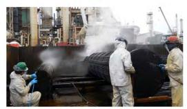
Hydro blasting & Pressure Washing All types of high pressure water cleaning: pumps from 15HP to 1,500HP with pressures from 2,500 PSI to 25,000 PSI. Experienced in heat exchangers/tube bundles, finfan coolers, clinker/ash removal, dewatering bins, all storage tanks, pipe/culvert cleaning.
