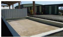
Secondary Containment Systems Customized spray or trowel-on coating systems to meet your chemical storage needs. All applications meet EPA requirements for containment of accidental spills. Proper surface preparation includes concrete repairs and sealants.
